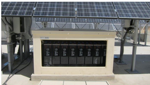
BATT'BOX with open front panel
